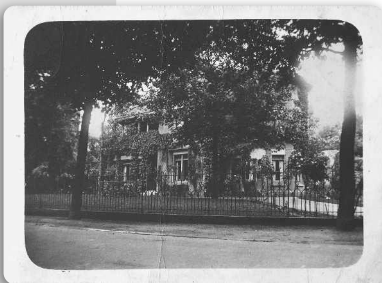
Eslaan 10, Villa Tsjido, architect H.P. Berlage, afgebroken
